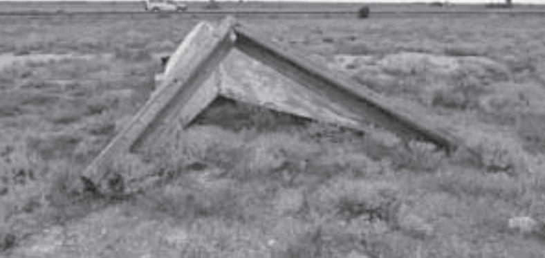
The peak of the collapsed northern monument at Ooldea
